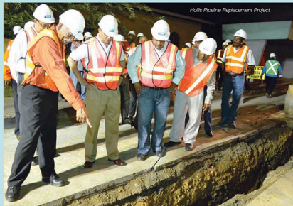
Holla Pipeline Replacement Project
